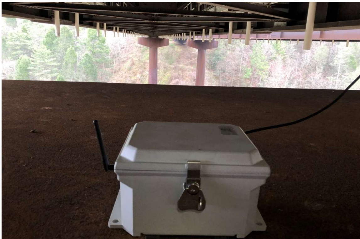
Figure 2. Sample Wireless Data Acquisition Gateway Attached to a Solar Panel (Not Shown)
