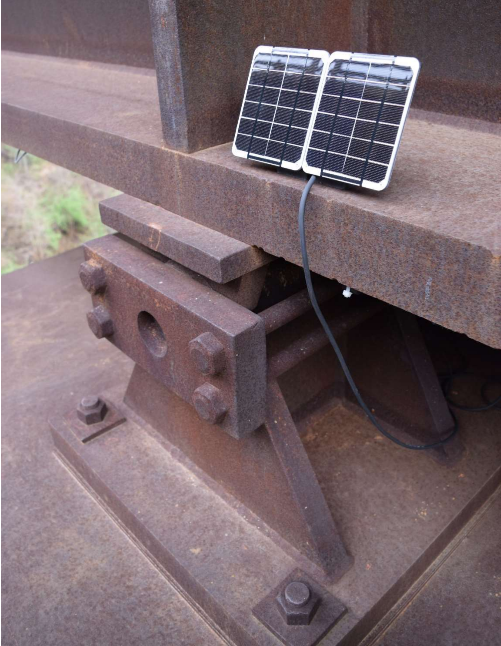
Figure 3. Sample Solar Panel for Wireless Data Acquisition Gateway (Not Shown)
